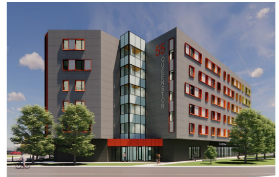
Image courtesy of Invizij Architects
