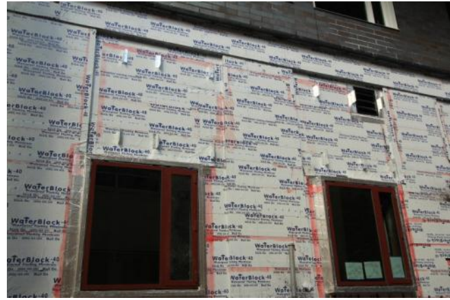
Fig.2.19 Self-Adhered Membrane (SAM) Air Barrier Membrane Applied to Fiberglass Faced Gypsum Sheathing. The simplicity of this system and use of exterior insulation makes this air barrier system common for non-combustible high-rise MURB construction and in particularly for exterior enclosure rehabilitations.
