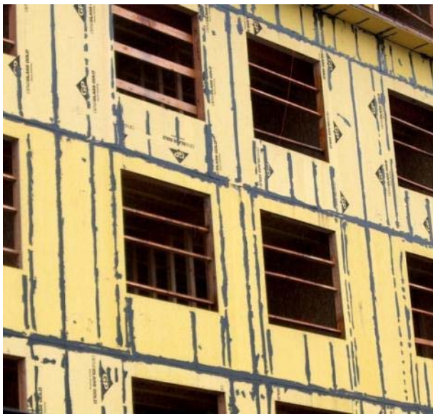
Fig.2.14 Sealed Sheathing Approach. This approach utilizes the rigid exterior sheathing sealed with sealants, membranes or tapes. The system provides good performance for all MURB heights due to rigidity, ease of inspection and detailing.
