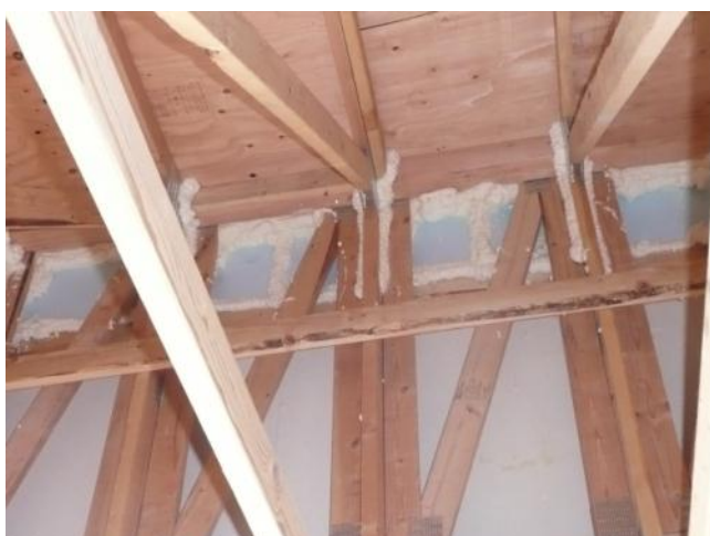
Fig.2.21 Sprayfoam used as transition material as part of other air barrier strategies. Sprayfoam is often used between floor and roof joists for continuity between wall and roof elements. In some cases, where the sprayfoam is poorly applied, touch-ups are needed to seal cracks and gaps missed during the first pass.
