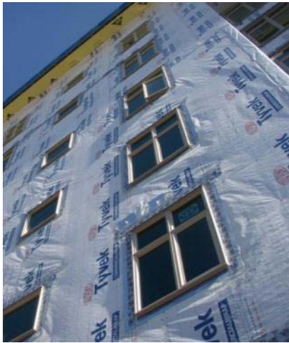
Fig.2.15 Sealed Sheathing Membrane Air Barrier Approach. When properly detailed and supported, the sealed exterior sheathing membrane air barrier approach can be a successful strategy for airflow control in a MURB. Notice the use of tapes to seal the sheathing membrane for this 4-storey wood-frame MURB. Rigidity and support of the membrane will be added in form of vertical wood strapping used to create the cavity for a rainscreen wall assembly.
