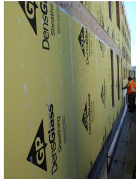
Fig.2.14 Sealed Sheathing Approach. This approach utilizes the rigid exterior sheathing sealed with sealants, membranes or tapes. The system provides good performance for all MURB heights due to rigidity, ease of inspection and detailing.
