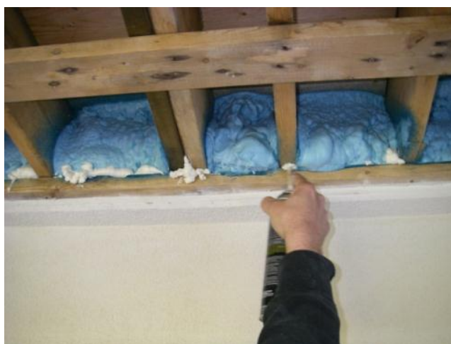
Fig.2.21 Sprayfoam used as transition material as part of other air barrier strategies. Sprayfoam is often used between floor and roof joists for continuity between wall and roof elements. In some cases, where the sprayfoam is poorly applied, touch-ups are needed to seal cracks and gaps missed during the first pass.
