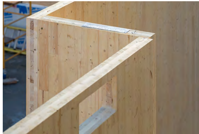
Figure 27 CLT wall panels with exposed penetrations and rough openings prior to on-site application of a WRB membrane.
