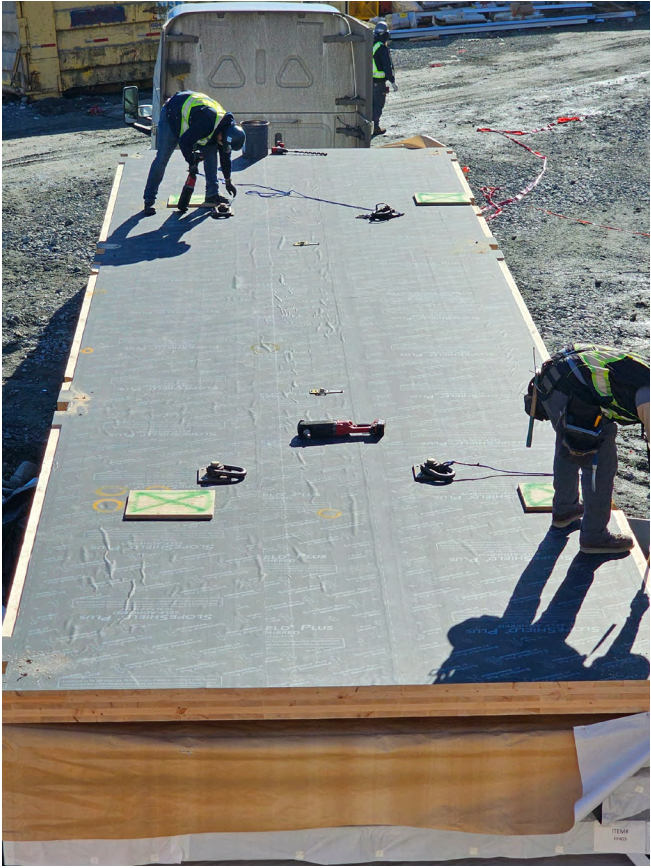
Figure 51 Panels are delivered to site and installed directly from the truck. The panels have a protection membrane installed to the face of the timber.
