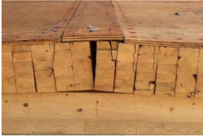
f) Built-up timber panel damage and distortion resulting from moisture-related panel expansion.
