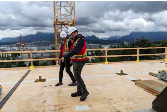
Figure 63 Visual inspection of mass timber floor during the construction phase to identify areas of damaged membrane, trapped water, etc.
