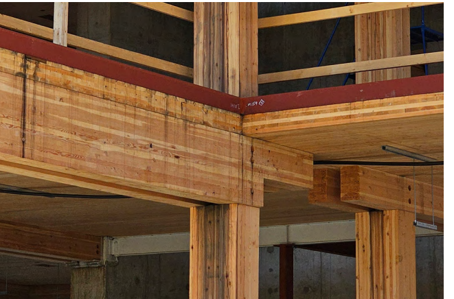
Figure 73 An example of staining caused by a reaction between iron and wood tannins in a mass timber project exposed to wetting from above.
