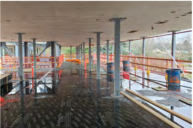
Figure 10 A mass timber floor exposed to rainwater during construction. A membrane is installed over full panels to reduce moisture-related risks.
