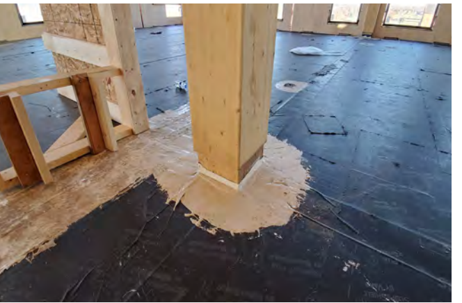
Figure 58 A temporary column detail that prevents water from traveling into the column connection.
