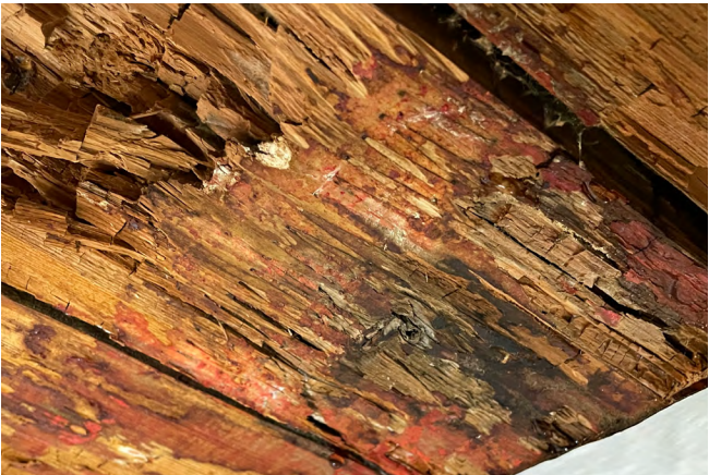
i) Severe deterioration of a CLT floor/soffit condition due to water intrusion from the wall above and the use of low-permeance membranes on both the top and bottom of the floor panel.
