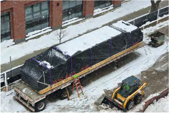
Figure 52 A mass timber panel is transported to the construction site on a truck bed. The mass timber is completely covered in a secure, heavy-duty tarp.
