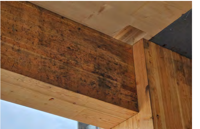
Figure 50 Mass timber beam with discolorations caused by staining from iron filings.
