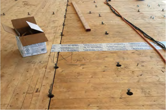
Figure 22 Timber-concrete composite CLT floor with shear connectors installed prior to concrete pour.
