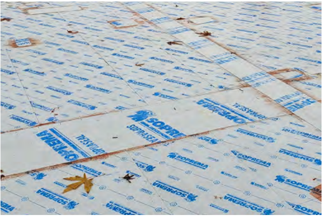
e) Vapor-impermeable self-adhered membrane.
