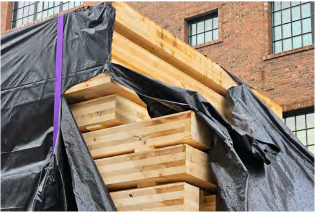
Figure 53 CLT panels covered in plastic when stored on-site. The plastic was not durable and not secured, leading to the exposure and wetting of the stored panels.
