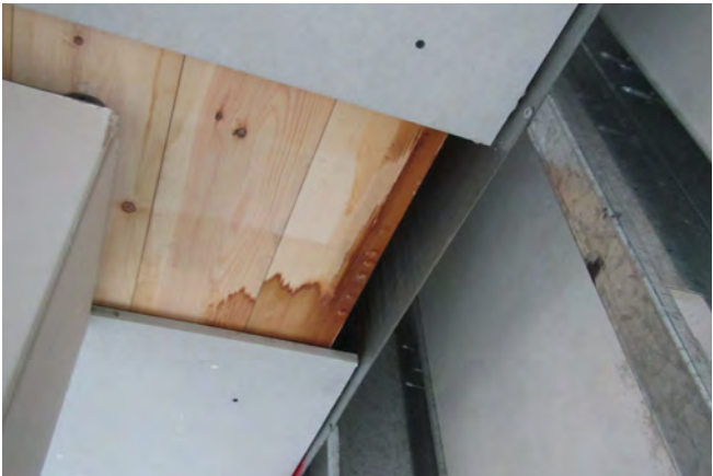
b) Moisture accumulation within a mass timber ceiling cavity due to the installation of interior gypsum board before the installation of adequate moisture protection on the floor panel above.
