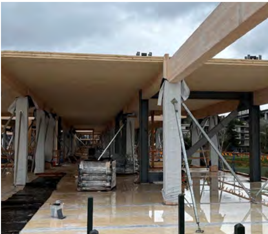
Figure 82 The protective membrane provided protection to the CLT and glulam even in very wet conditions.
