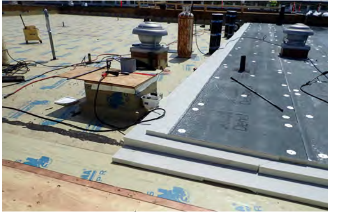
Figure 17 A roof assembly with mechanically fastened insulation and coverboard system. The fasteners are installed through the membrane, which acts as the construction phase moisture protection and the permanent air and vapor barrier.
