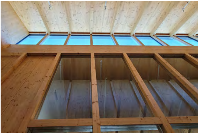
Figure 75 The underside of a mass timber roof and exterior windows that are a part of the building enclosure.
