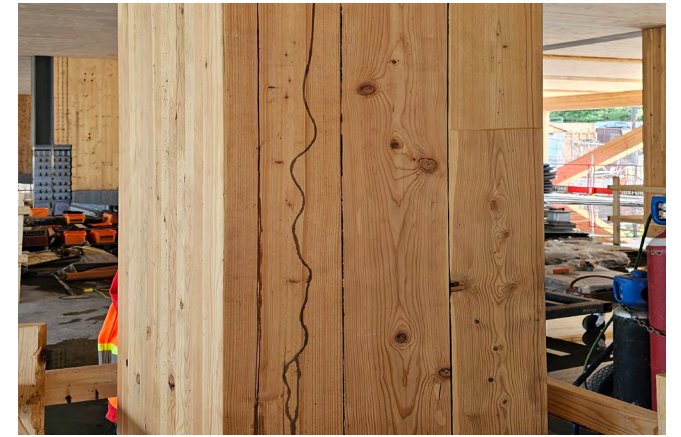
Figure 29 A glulam column with dark iron staining from water traveling down the column from the level above.
