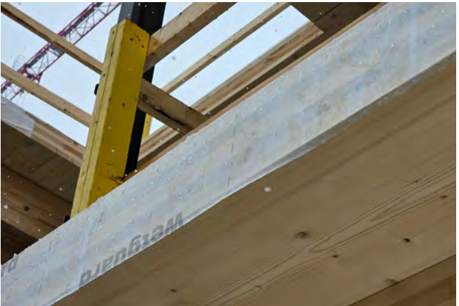
Figure 11 A protective membrane is installed over the end grain at the perimeter of a CLT floor to reduce moisture-related risks.
