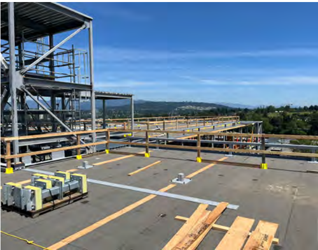
Figure 45 Factory-applied roofing base sheet moisture protection over CLT at the roof level.
