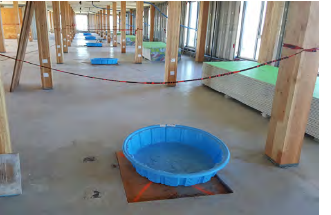
h) Water collection with kiddie pools (other collection devices like pails can also be used). The collected water is regularly removed from the building.
