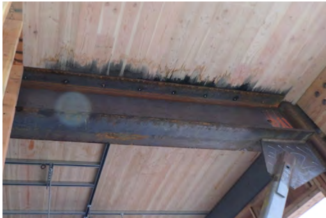
d) Visible staining on the underside of a CLT floor panel due to the damp wood being in direct contact with unfinished steel, resulting in a chemical reaction between the wood tannins and metal.
