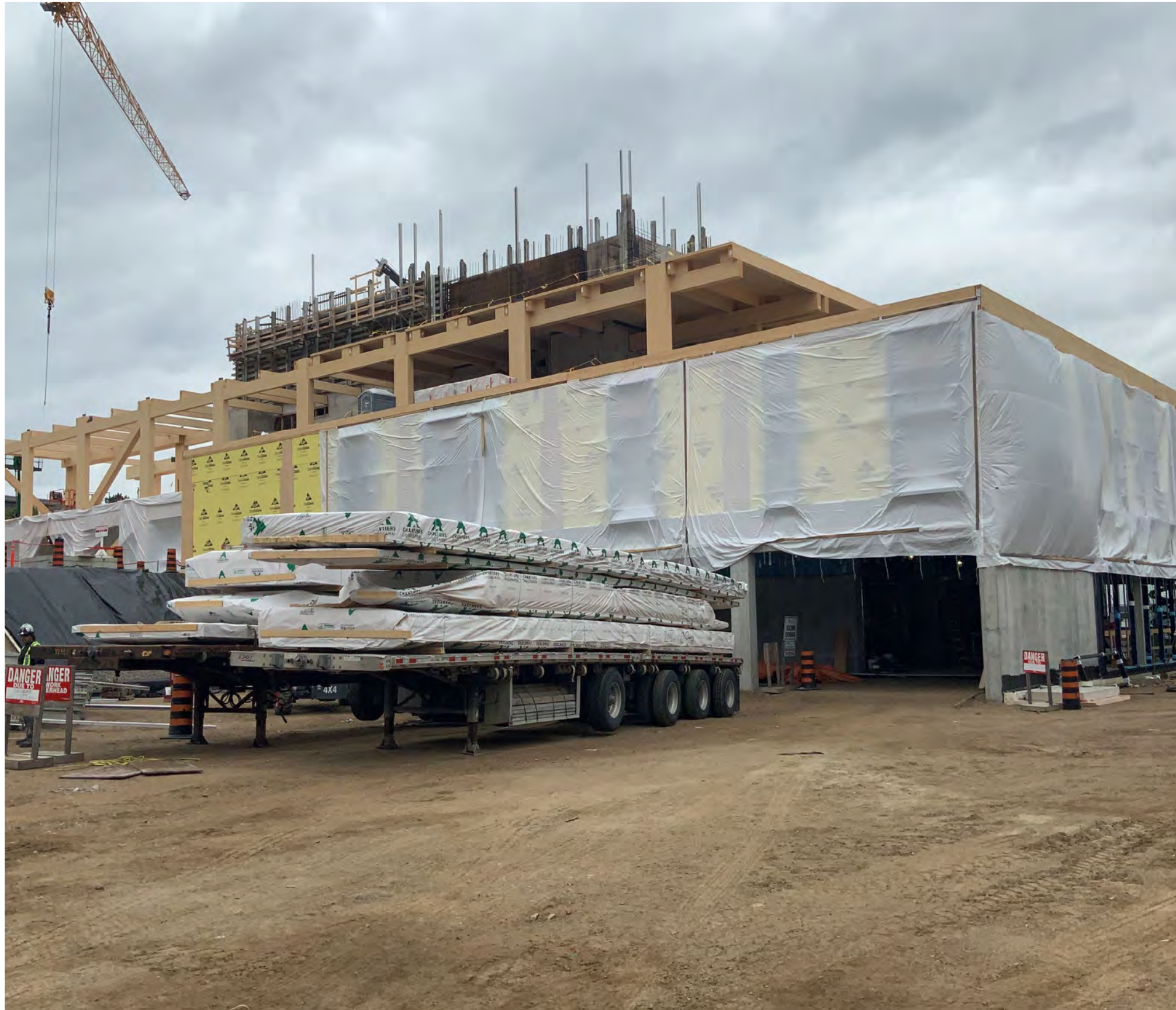
Figure 41 Mid-construction of the mass timber Science Collaboration Centre in Chalk River, Ontario. Perimeter hoarding is installed as each floor is completed to protect the mass timber from moisture exposure (Canadian Nuclear Laboratories).
