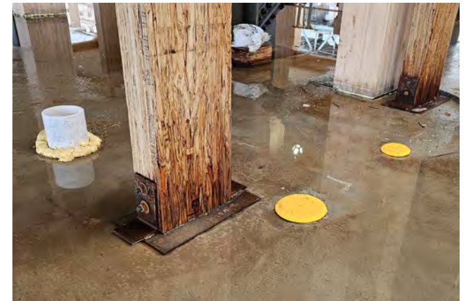
Figure 31 Water absorption at the base of a parallel strand lumber (PSL) column due to contact with wet surface conditions.
