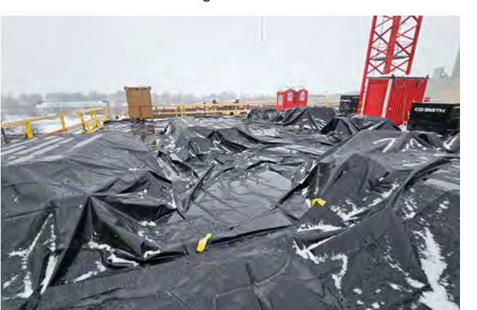
i) A tarp used to collect snow, which is then removed from the building using the overhead crane.
