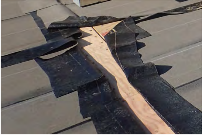
Figure 13 A mass timber roof assembly. Once all laps of the membrane are sealed, the air and vapor barrier membrane visible in this photo will temporarily protect the mass timber from moisture (Catalyst, Spokane, WA).
