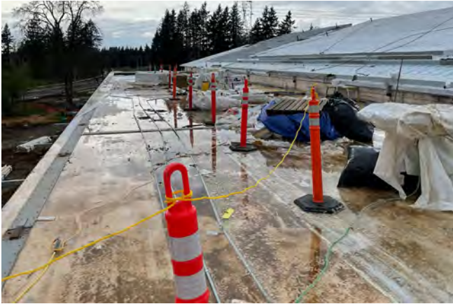
Figure 61 Mass timber roof where ponding water is not being removed. Water has gotten underneath the protective membrane through laps and areas of damage to the membrane, resulting in wet mass timber and staining.
