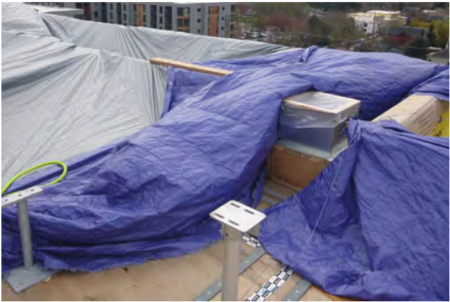
Figure 54 A tarp installed over the mass timber parapet at a roof has left a portion of the roof exposed and at risk of wind-driven rain migrating under the edges of the tarp. Water is not able to drain from the tarp, so removal with shop vacuums or pumps is required.
