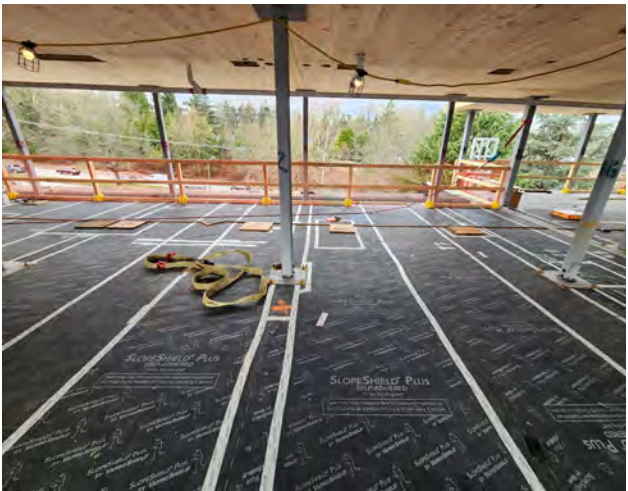
Figure 44 Factory-applied vapor-permeable moisture protection membrane over CLT at the intermediate floor level.
