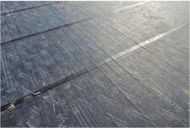
d) Vapor-permeable self-adhered membrane.
