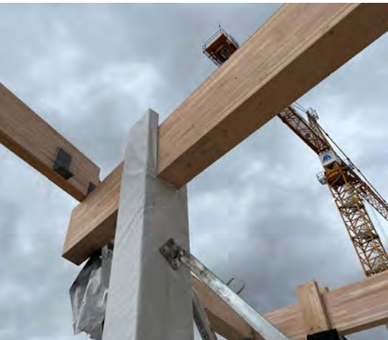
Figure 81 Glulam beams during construction.
