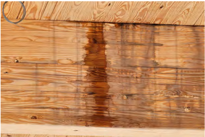
c) Staining on a CLT wall and intermediate floor panels due to ponding water on the floor panels above.
