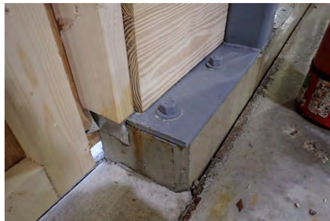
Figure 28 A CLT wall is installed onto a concrete curb to elevate the base of wall above grade level. The CLT and concrete curb are separated with a metal attachment.
