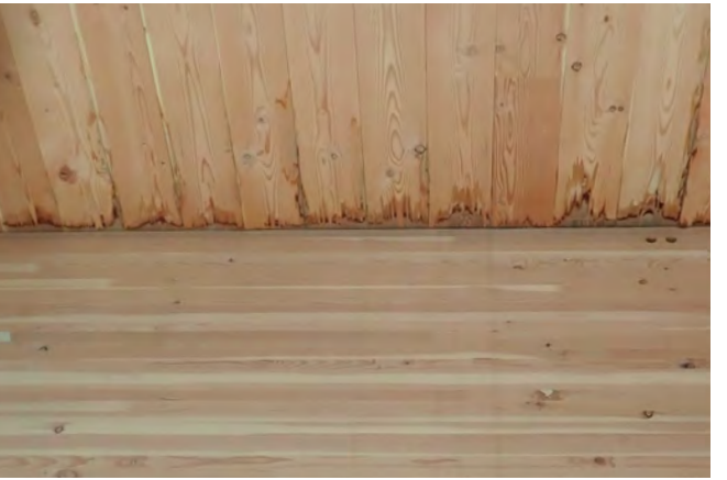
Figure 72 An example of general wood staining caused by wood tannins migrating with the water in a mass timber project exposed to wetting from above.
