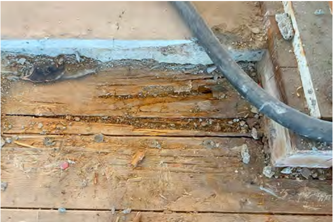
Figure 7 A CLT floor with concrete topping removed to reveal decay of the wood.
