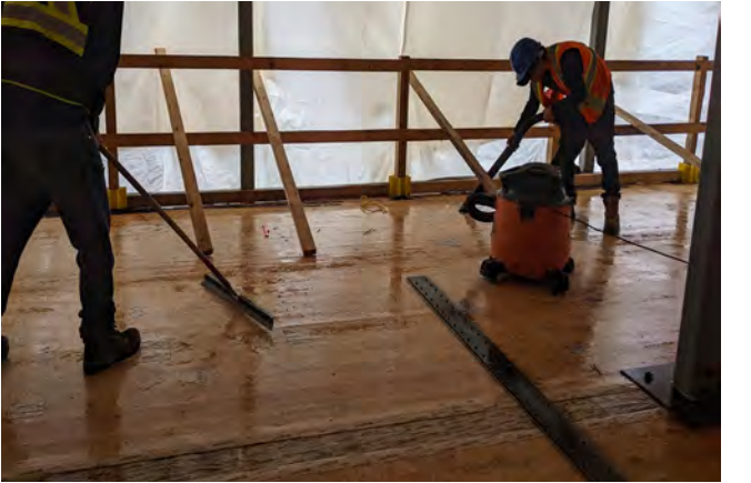
Figure 48 An on-site crew is mobilized to remove water from a mass timber floor using squeegees and shop vacuums.
