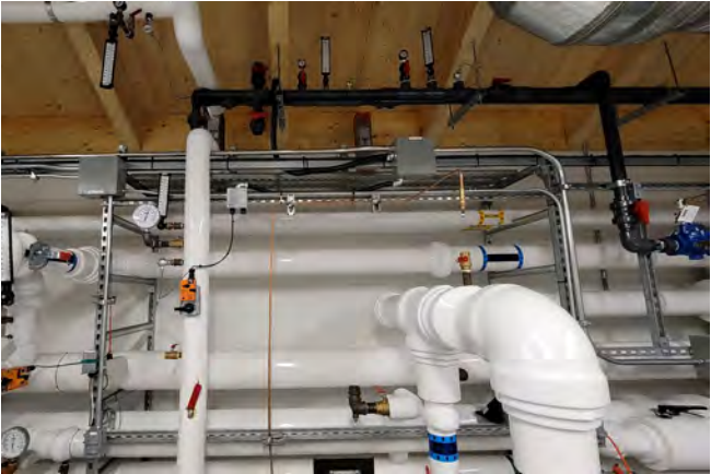
Figure 36 A mechanical room in a mass timber building. Installing targeted moisture protection at the mechanical room floor assembly, and regular inspection and maintenance of the equipment and piping, is recommended to reduce the risk of wetting the mass timber during occupancy.
