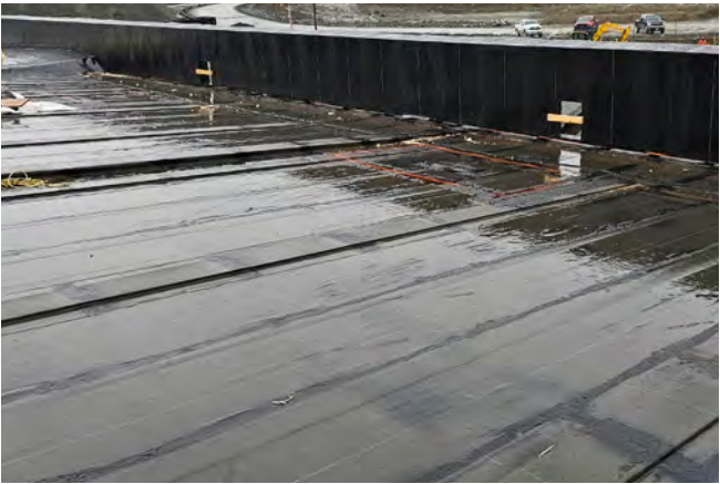
f) Vapor-impermeable self-adhered SBS roofing base sheet.
