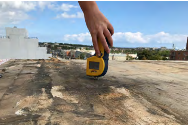
h) Microbial growth and deterioration of an unprotected CLT roof panel.
