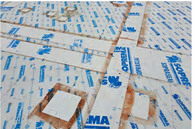
Figure 59 A mass timber roof where the protective membranes were regularly repaired and patched. Membrane patches and strips were installed over panel joints, areas of damage, and structural steel connections.
