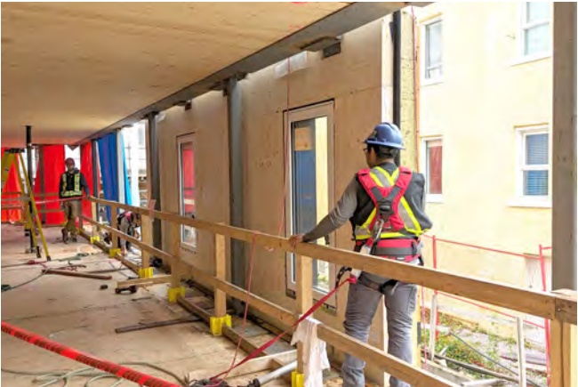
Figure 8 A mass timber building with prefabricated wall panels being installed prior to concrete topping placement.
