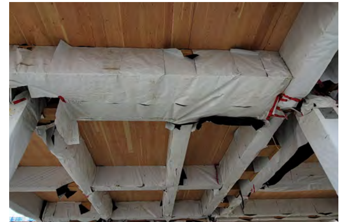
Figure 30 Glulam columns and beams protected using the factory wrapping. The factory wrapping is removed at structural connection, and the wrapping at the underside of beams and bottom of the column is opened to allow for water drainage.
