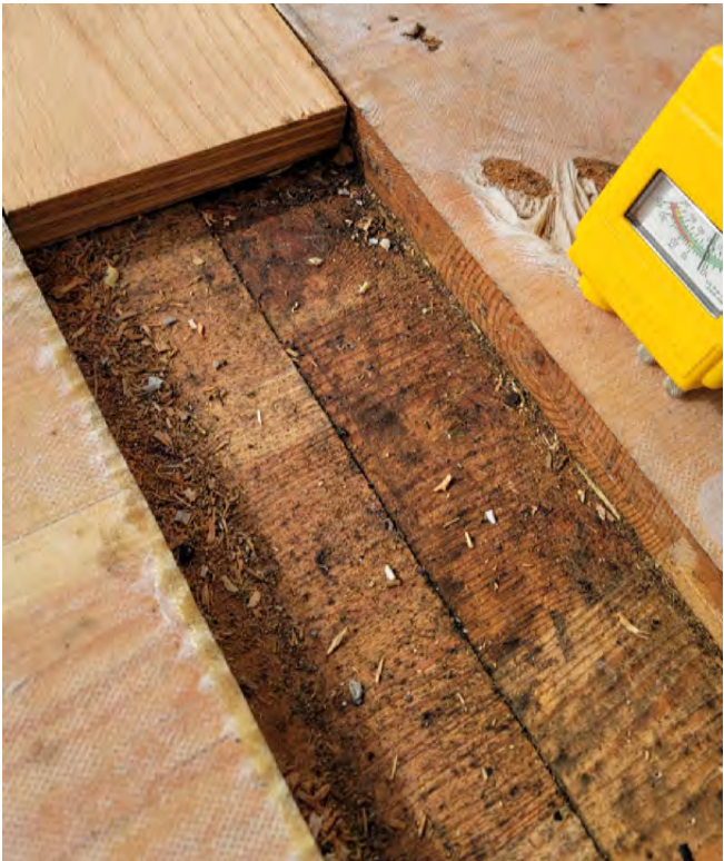
Figure 66 Mass timber joint with its spline removed and wet wood visible. Moisture was trapped undetected under the spline.
