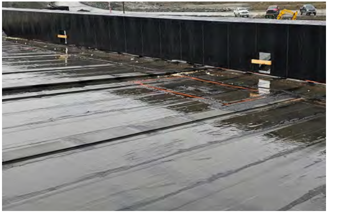
Figure 16 A sloped CLT roof panel with a vapor-impermeable roofing base sheet acting as the moisture protection membrane during construction. The membrane will act as the base ply of the final 2-ply roof membrane. The panel slopes to the roof perimeter.
