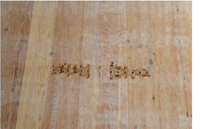
Figure 49 Holes in the protective membrane where a temporary fall protection anchor was installed. A membrane patch was not installed once the anchor was removed.
