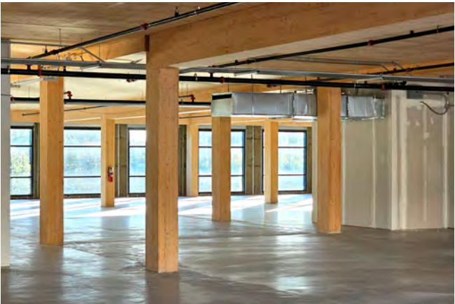
Figure 35 A fire suppression sprinkler system in a mass timber building. If the sprinkler system is used during occupancy, it will be necessary to identify locations where water may have traveled beneath the concrete topping.
